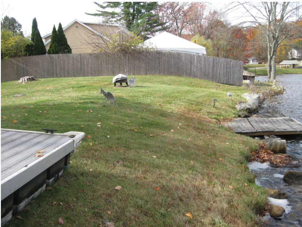
Photo No. 16: Dike on Lot 112 looking right toward the restaurant.
