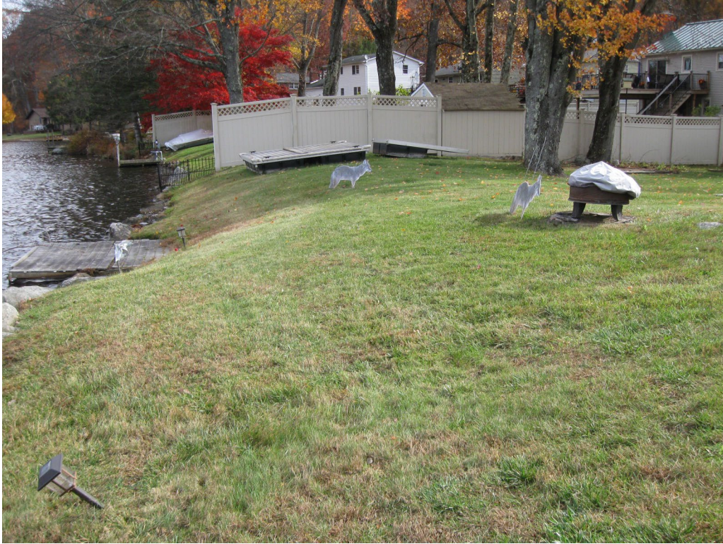
Photo No. 15: Dike on Lot 113 looking left.
