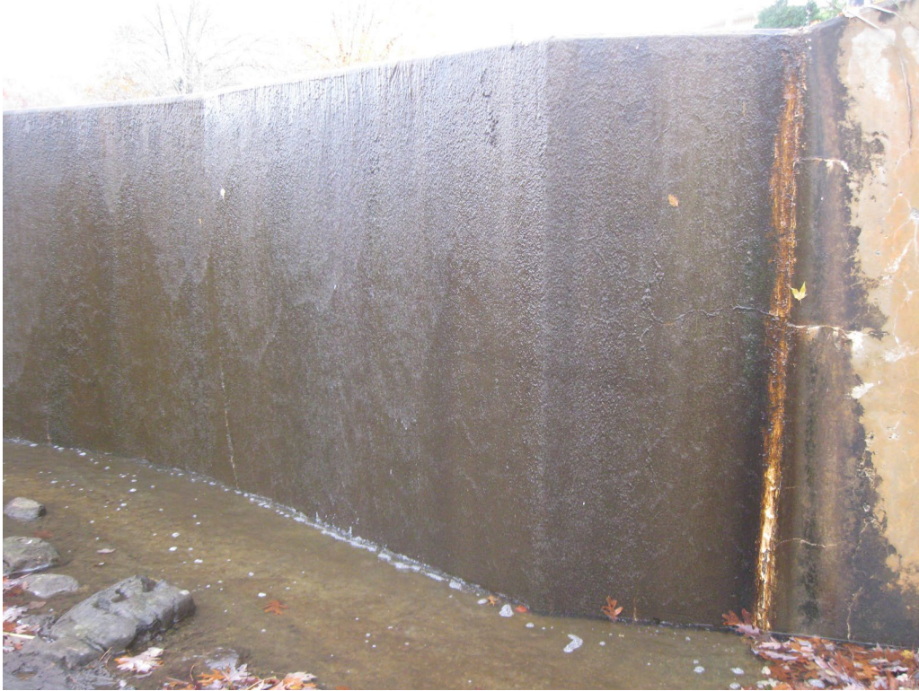
Photo No. 23: Left side downstream face of spillway.
