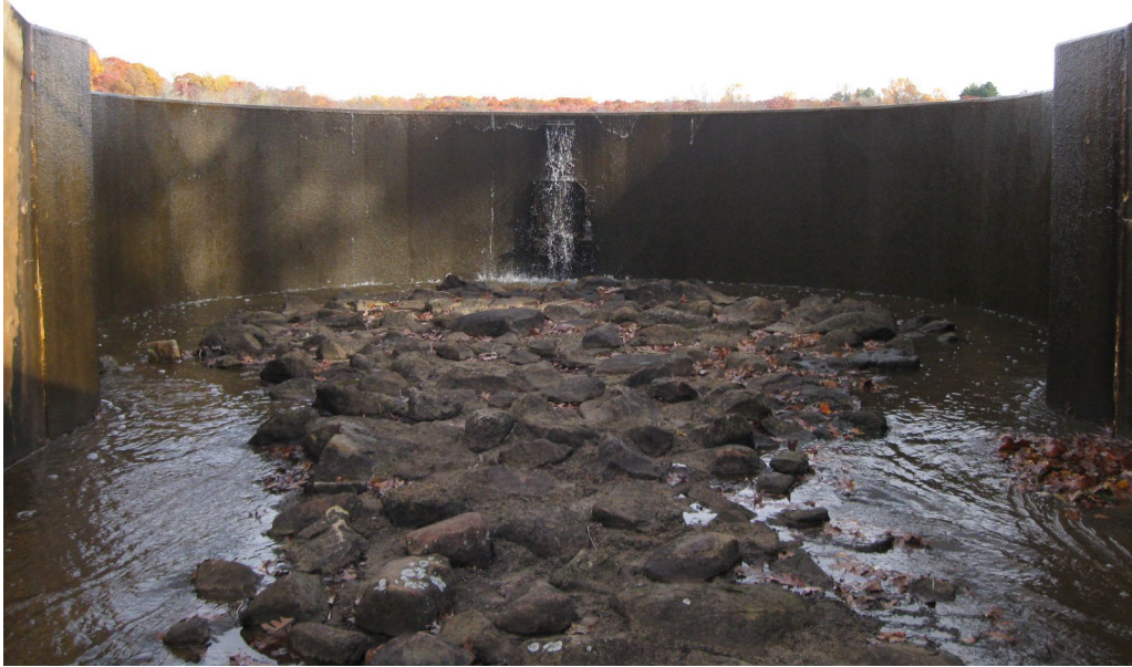
Photo No. 29: Spillway and grouted riprap discharge channel looking upstream.
