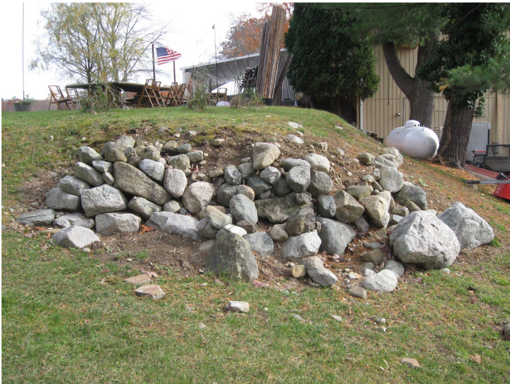
Photo No. 14: Closeup of the rock rubble wall on the left side downstream slope of the dam looking left toward the restaurant.
