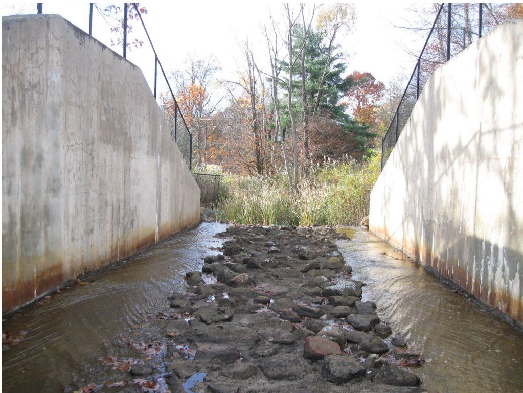
Photo No. 30: Grouted riprap discharge channel looking downstream.
