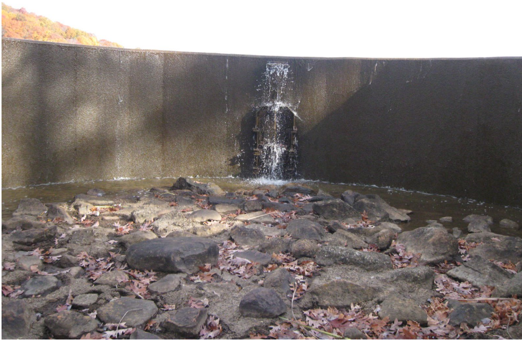
Photo No. 19: Downstream face of spillway looking upstream.
