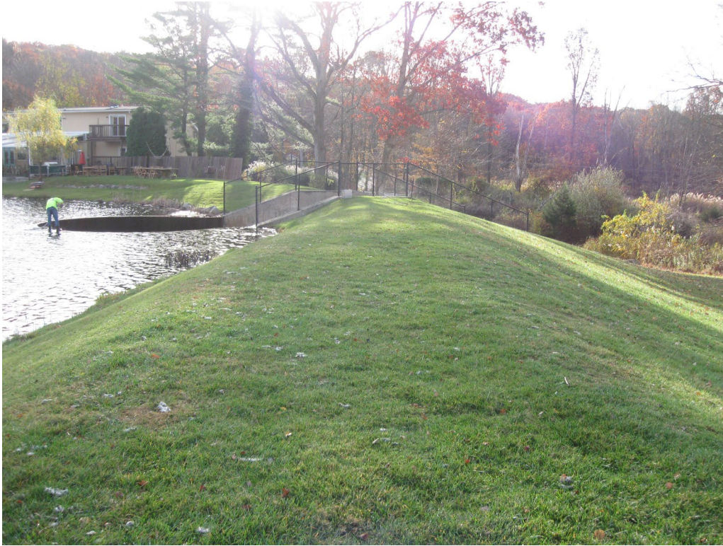
Photo No. 1: Right side dam crest looking left toward the spillway.
