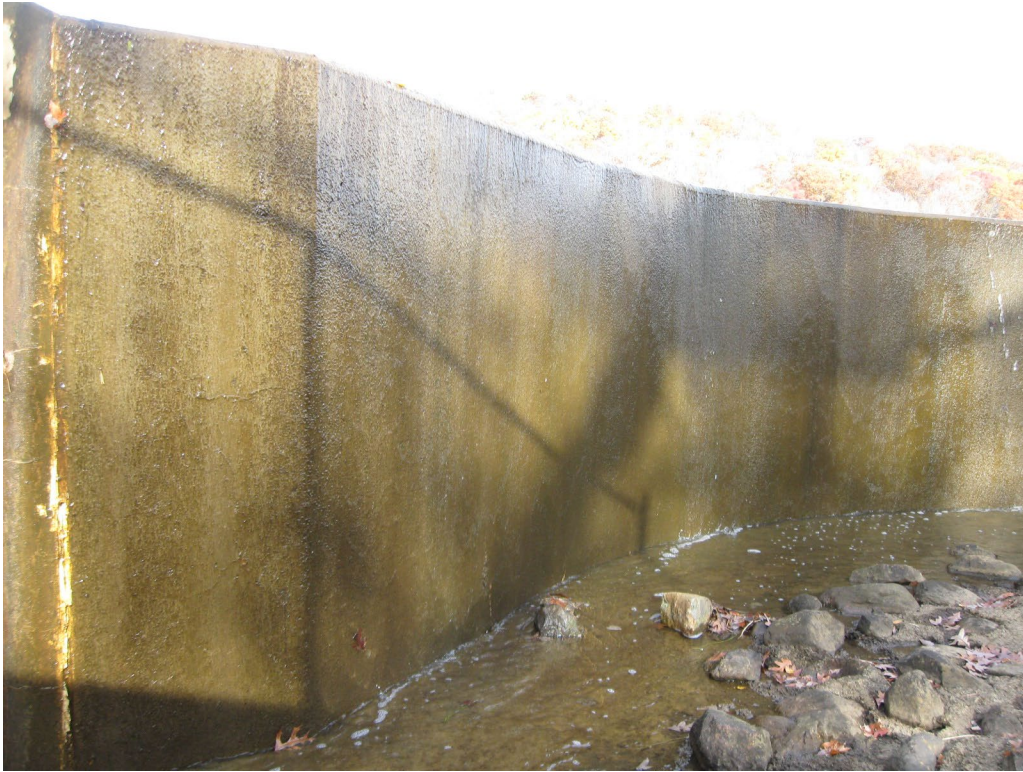
Photo No. 21: Right side downstream face of spillway.
