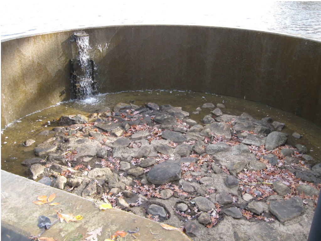
Photo No. 18: Downstream face of spillway looking left.
