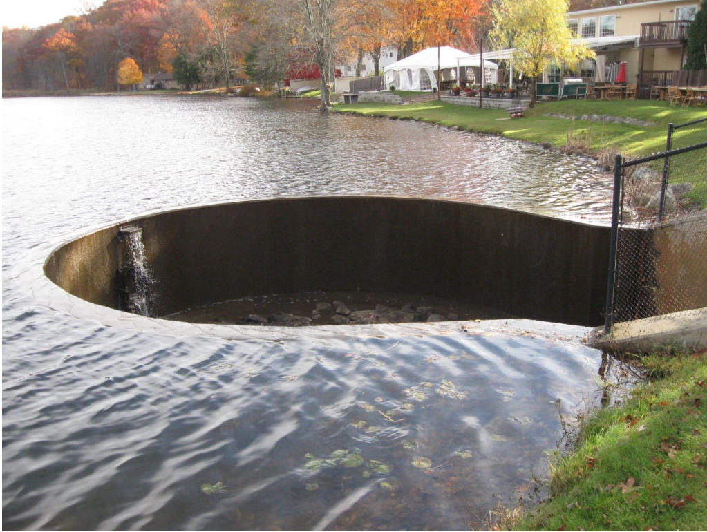
Photo No. 17: Spillway entrance and crest looking left.
