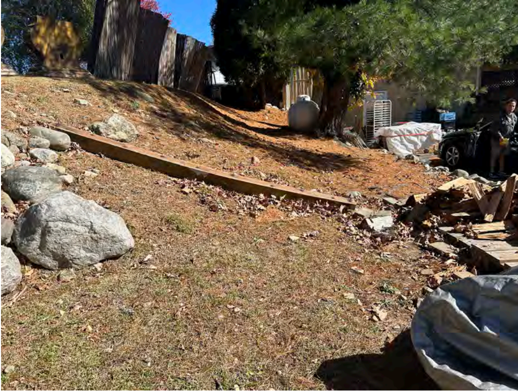
Photo No. 13: Left side downstream slope of the dam looking left toward the restaurant.
