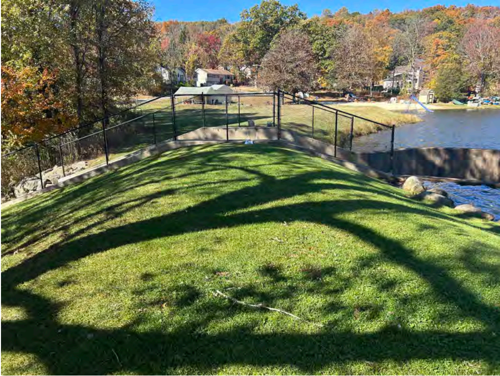
Photo No. 3: Left side dam crest looking right toward the spillway.
