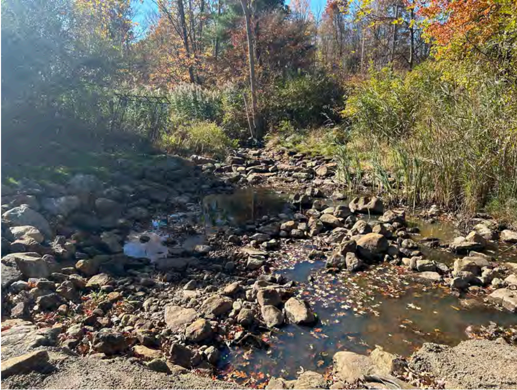
Photo No. 33: Looking downstream at the plunge pool and exit channel toward the Tomahawk Trail bridge.
