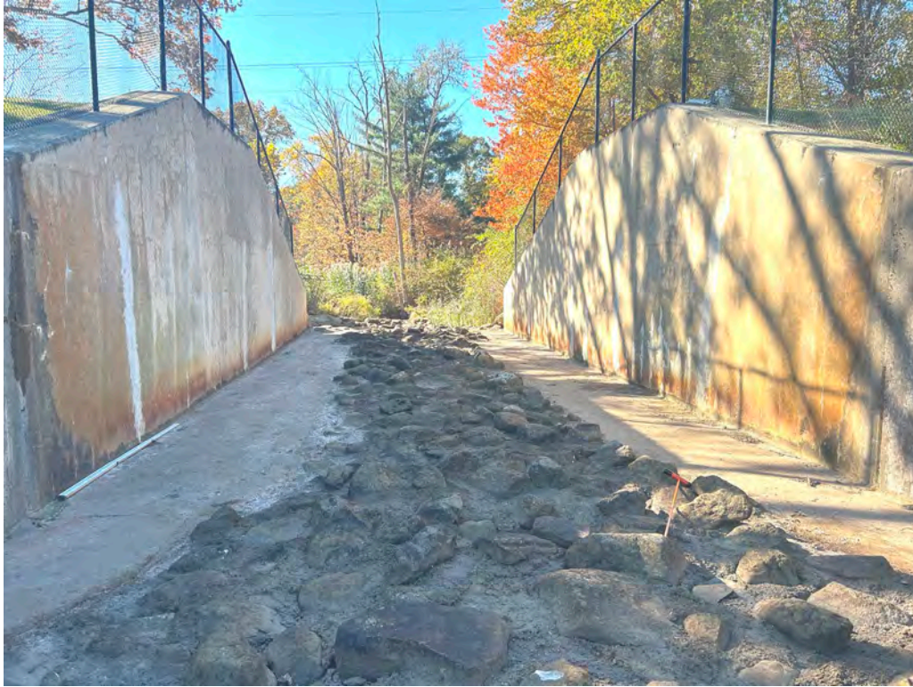
Photo No. 29: Grouted riprap discharge channel looking downstream.
