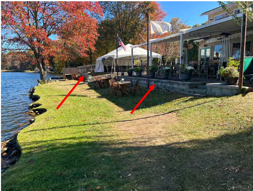
Photo No. 8: Left side upstream slope of the dam looking left along the restaurant. Note the segmental block retaining walls.
