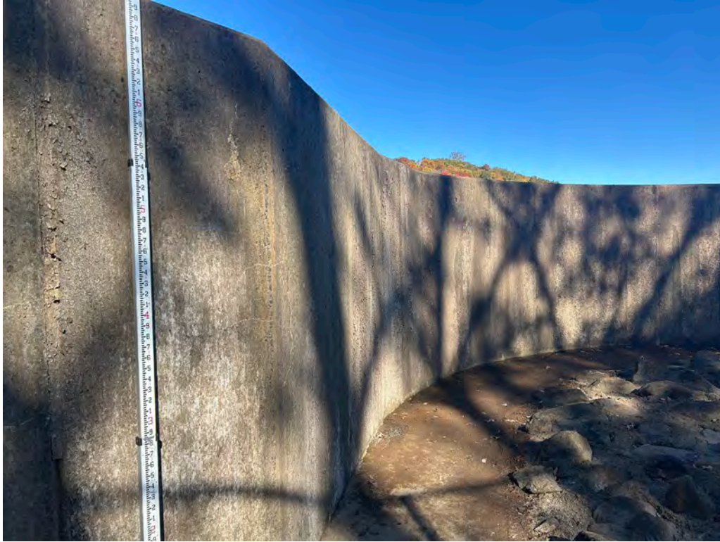
Photo No. 21: Right side downstream face of spillway looking upstream.
