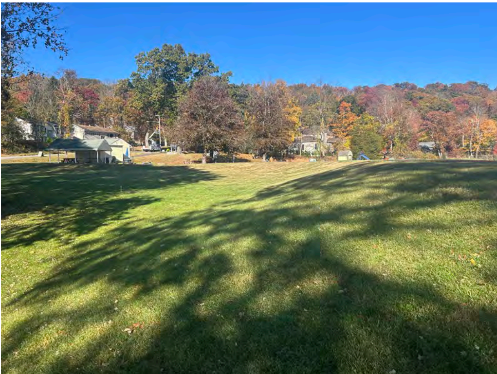
Photo No. 10: Right side downstream slope and toe of the dam looking right toward the right abutment.
