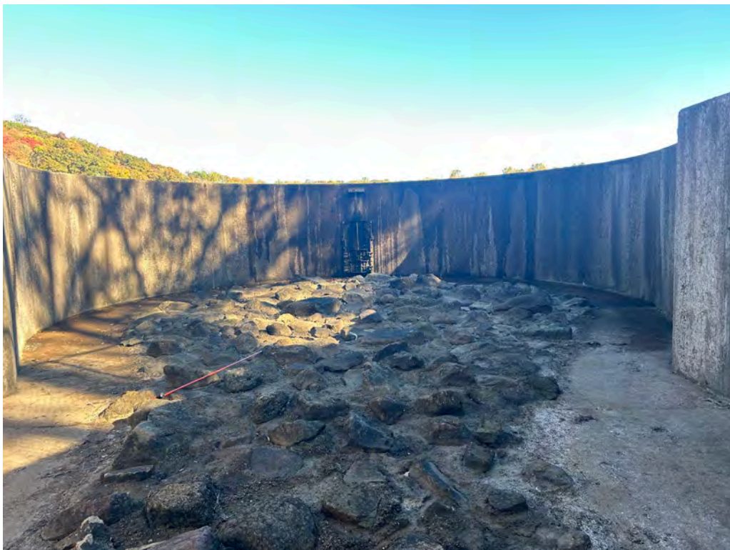
Photo No. 18: Downstream face of spillway looking upstream.
