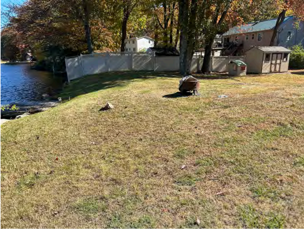
Photo No. 15: Dike on Lot 113 looking left.
