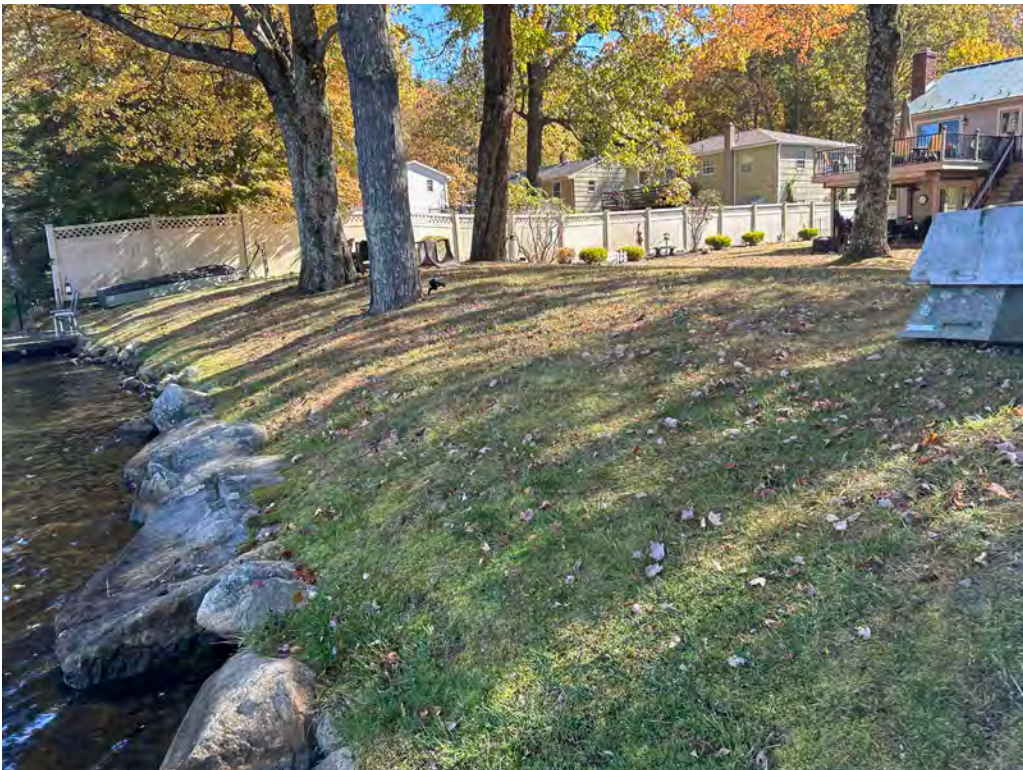
Photo No. 16: Dike on Lot 112 looking left.
