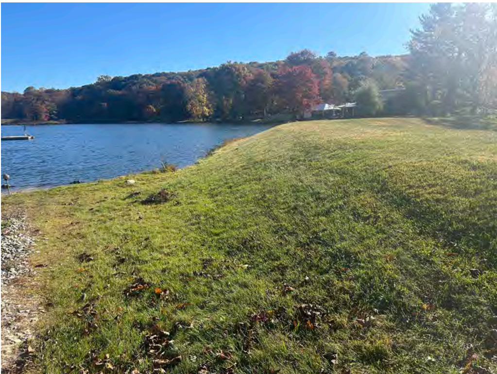
Photo No. 6: Right side upstream slope of the dam looking left toward the bend.
