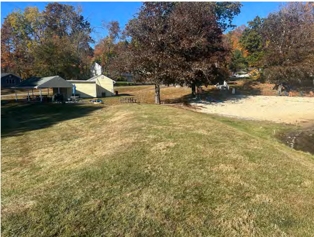
Photo No. 2: Right side dam crest looking right toward the right abutment.
