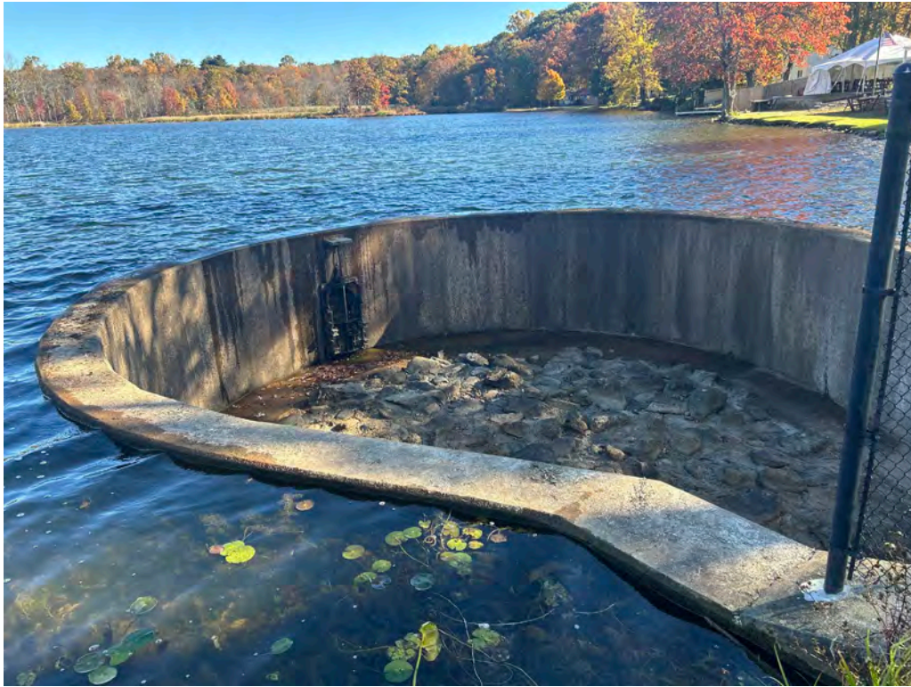
Photo No. 17: Spillway entrance, crest and downstream face looking left.
