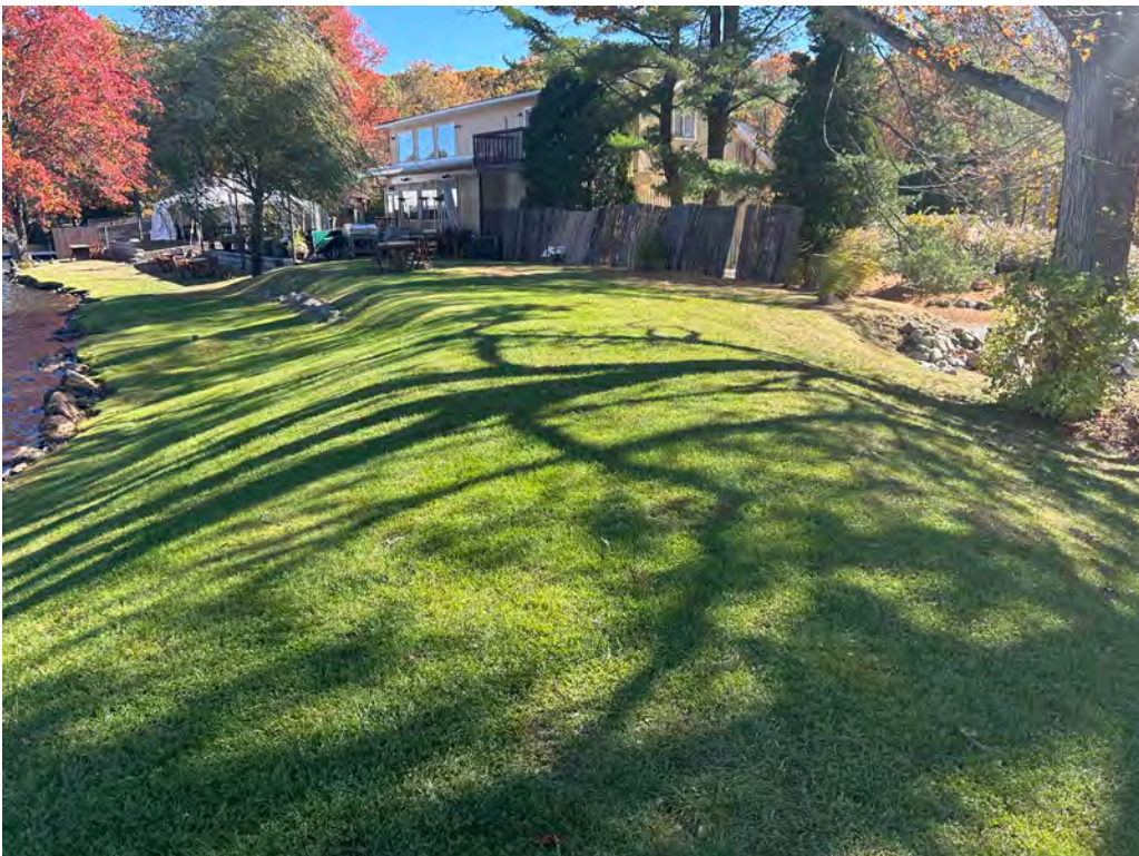
Photo No. 4: Left side dam crest looking left toward the restaurant and dike.
