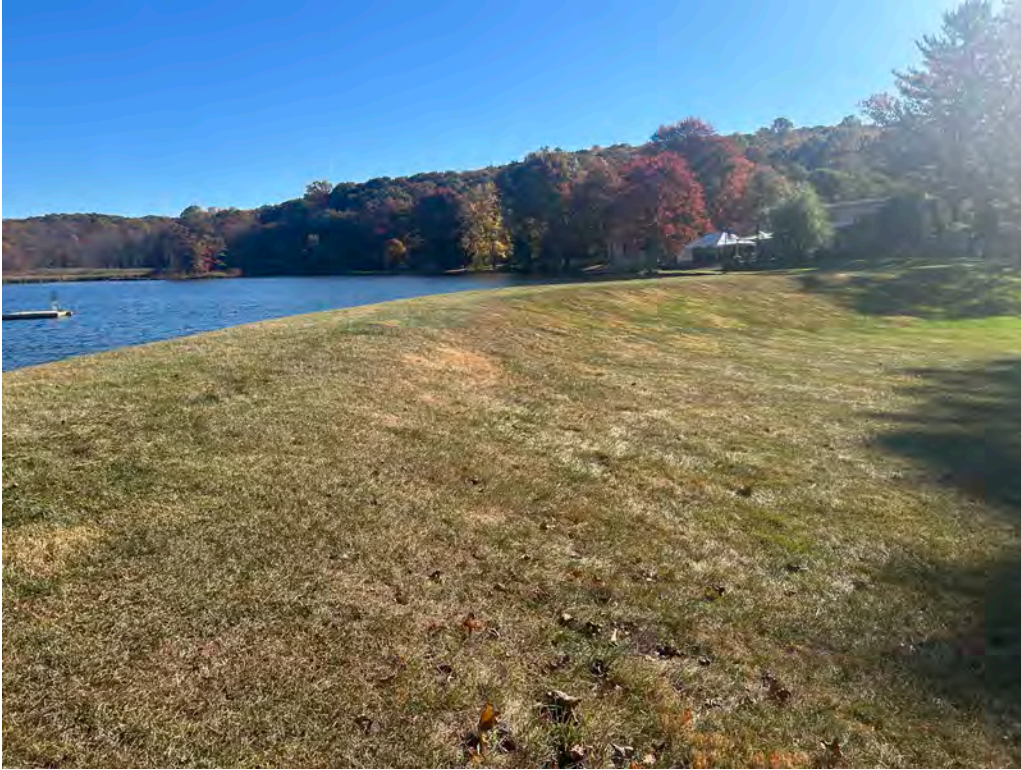
Photo No. 9: Right side downstream slope and toe of the dam looking left toward the spillway.
